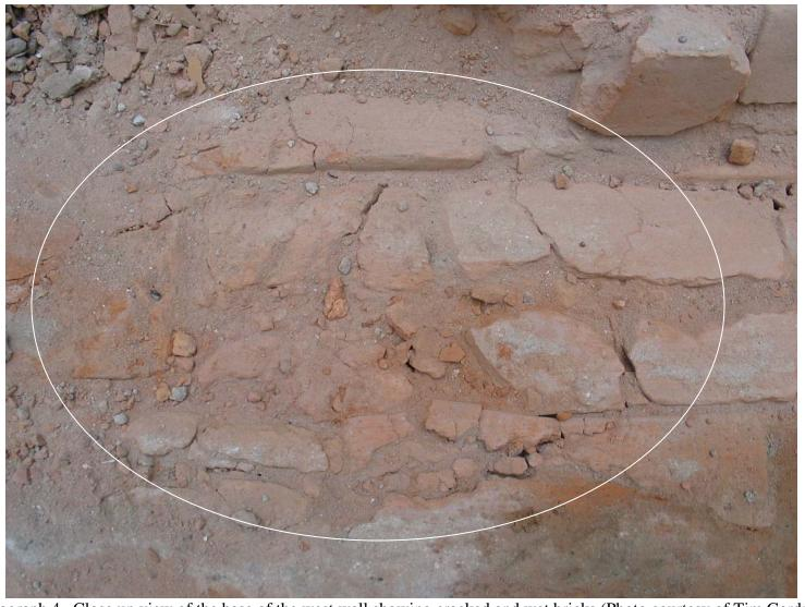
Photograph 4. Close up view of the base of the west wall showing cracked and wet bricks (Photo courtesy of Tim Gardner, Executive General Adjuster, Regional Manager, NHI General Adjusters)
