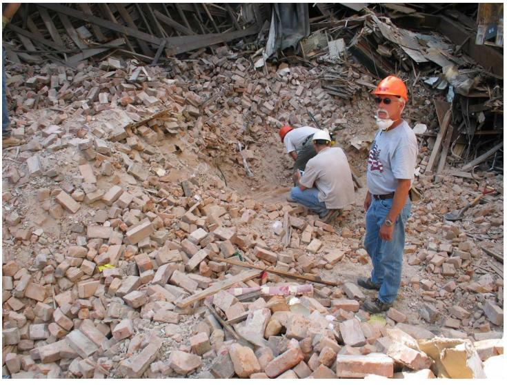
Photograph 2. Remnants of the west wall showing individual bricks, broken and pulverized (Note: no wall segments remained. Photo courtesy of Tim Gardner, Executive General Adjuster, Regional Manager, NHI General Adjusters)
