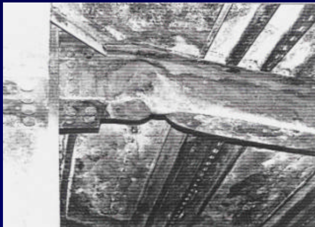
Beam Local Buckling
