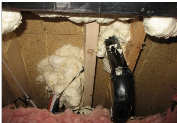
Drain and water lines after sealing
