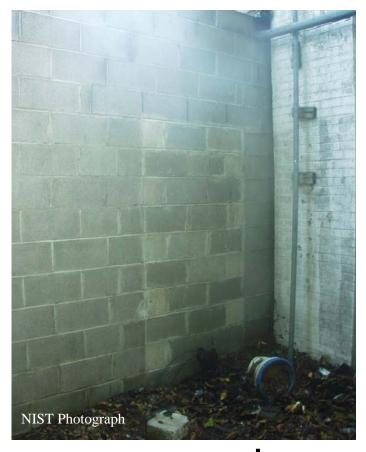
Figure I-5. Doorway on the rear wall of main showroom that was filled in with concrete blocks.
