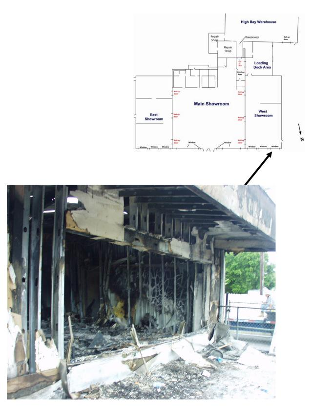
Figure E-3. Exterior view of front of west showroom. Metal stud walls visible.
