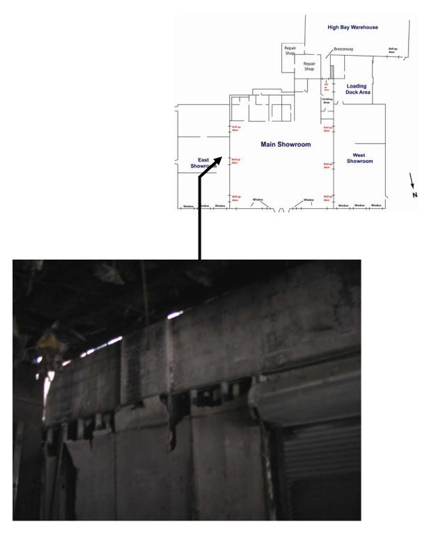
Figure F-20. Interior view of east showroom looking toward main showroom. Concrete block wall was originally exterior wall of grocery store. Gypsum wall board attached to metal stud which were attached to concrete block wall. Metal studs/gypsum wall board extended up to drop ceiling, but not above drop ceiling.
