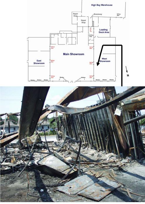
Figure E-29. Interior of west showroom along east wall toward front of store. Open roll-up fire door visible at right of photo.
