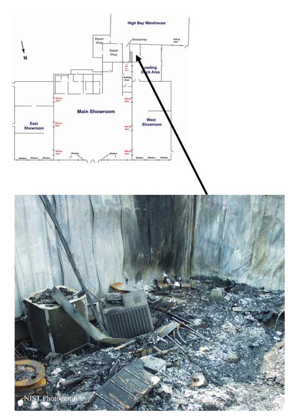
Figure C-18. Intersection of breezeway wall and north wall of warehouse. Heat pumps were located in small courtyard area between loading dock and breezeway wall. Gallon containers of hydrocarbon solvent can be seen at base of breezeway wall.
