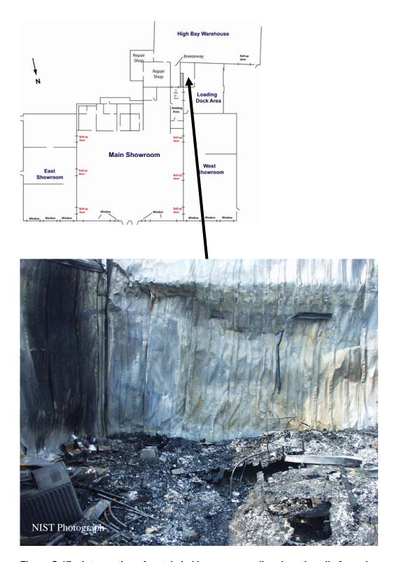
Figure C-17. Intersection of metal clad breezeway wall and north wall of warehouse.
