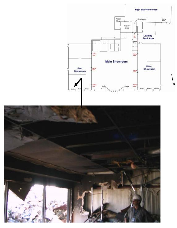
Figure F-17. Interior view of east showroom looking at drop ceiling. Exterior metal siding visible in center right of photo. Portions of gypsum wall board visible in center background of photo.
