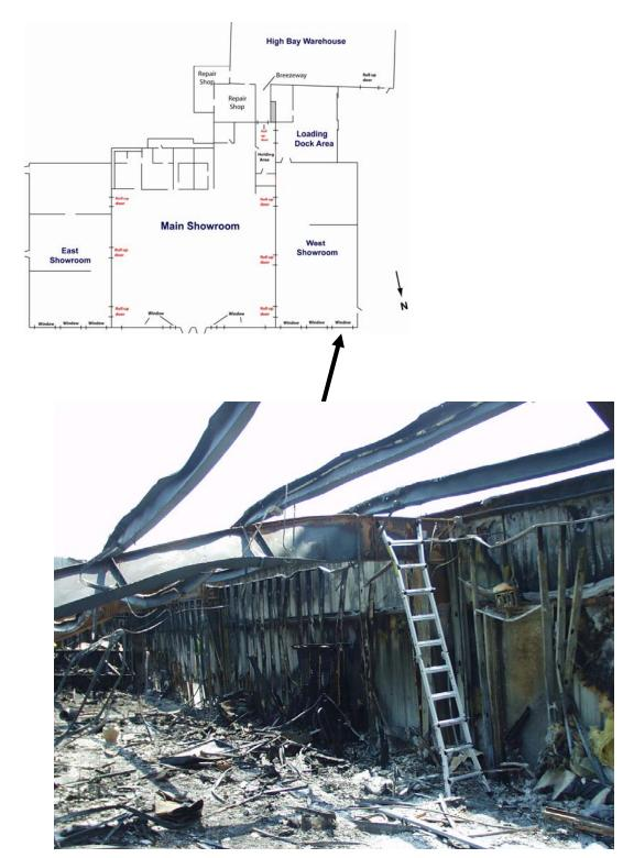
Figure E-17. Interior view of north-west corner of west showroom. Sagging I-beam and roof Z-channel visible in photo. Exit door in west wall near front of showroom visible to right of ladder.
