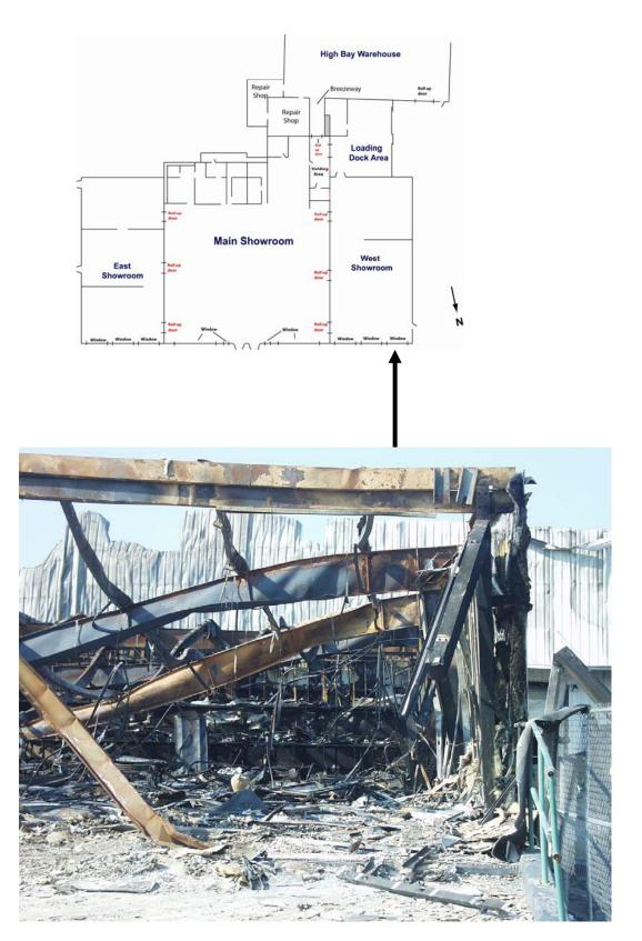
Figure E-10. Northwest corner of west showroom after removal of façade and roof.
