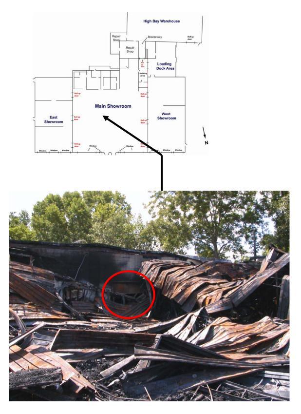
Figure D-24. Interior of main showroom looking toward east wall. Partially closed roll-up fire door circled.
