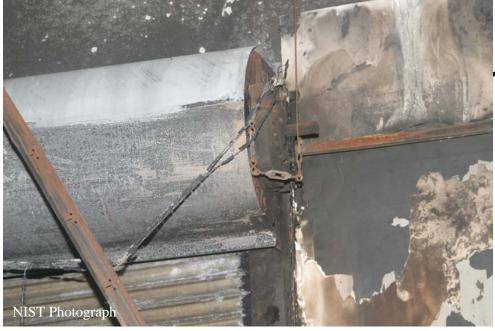
Figure O-34. North side of operating mechanism for roll-up fire door #5.
