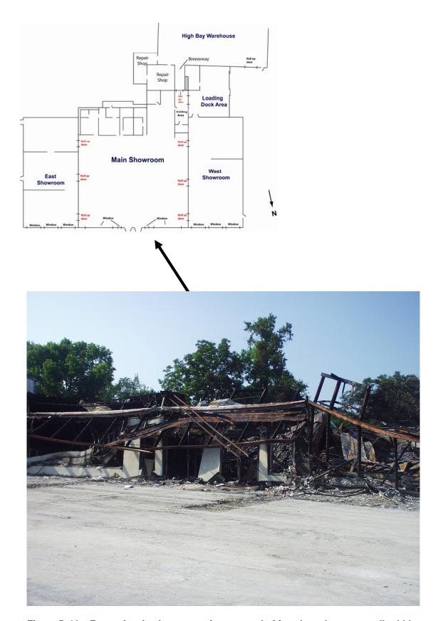
Figure D-12. Front of main showroom after removal of façade and parapet wall rubble.
