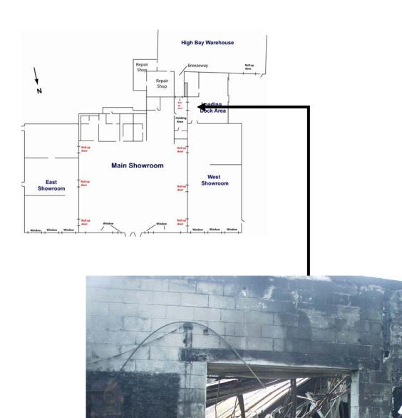
Figure C-9. Non-fire roll-up door between loading dock and holding area as viewed from loading dock.
