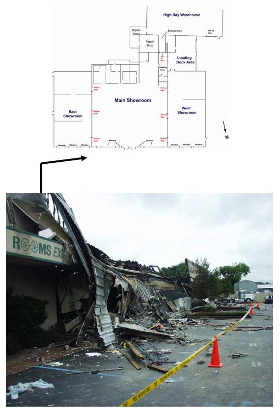
Figure D-3. Front of main showroom. Facade and parapet wall collapsed into parking spaces.
