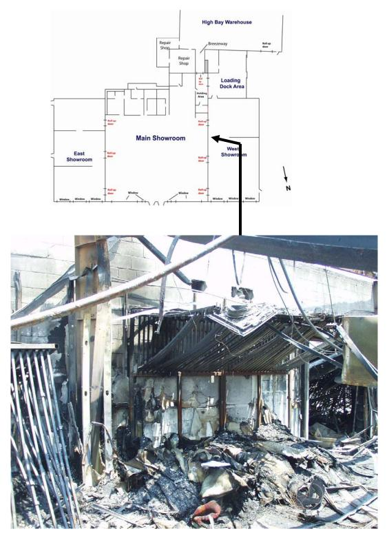
Figure E-25. Area rug support racks in west showroom. Open roll-up fire door visible on right of photo.
