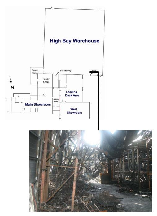
Figure G-15. Interior of warehouse looking from roll-up door toward repair shop doorway.
