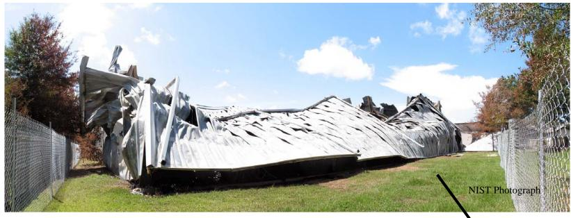
Figure B-19. East and south walls of warehouse looking towards loading dock.
