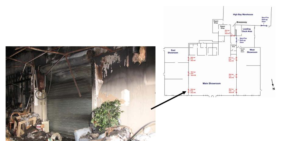
Figure O-33. Main showroom roll-up fire door looking toward front of main showroom. Door identified as roll-up fire door #5 in Figure O-1.
