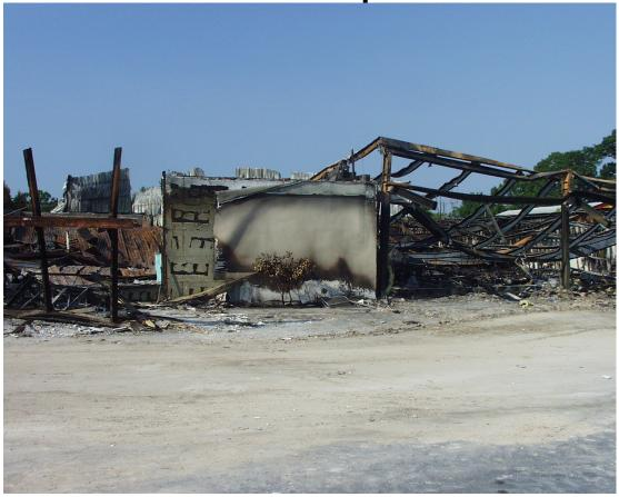
Figure E-15. Exterior view of front walls of main and west showrooms. Solid wall of main showroom is visible in center of photo.
