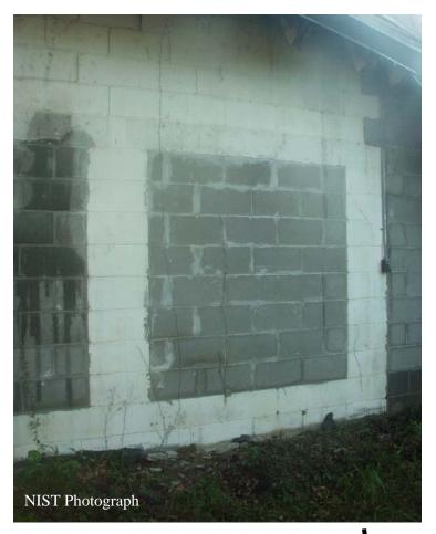
Figure I-9. Openings on the rear wall of main showroom that were filled in with concrete blocks.
