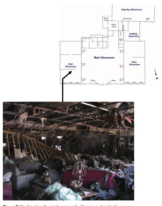
Figure F-14. Interior of east showroom looking toward main showroom. Closed roll-up fire door visible in center-right background. Partially closed roll-up fire door visible in center background. Photo displays less fire damage to furniture in front section of east showroom.
