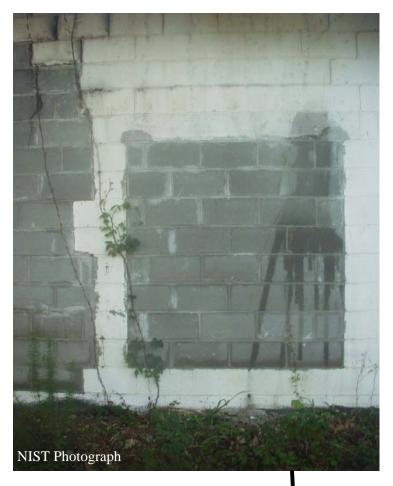
Figure I-10. Opening on the rear wall of main showroom that was filled in with concrete blocks.
