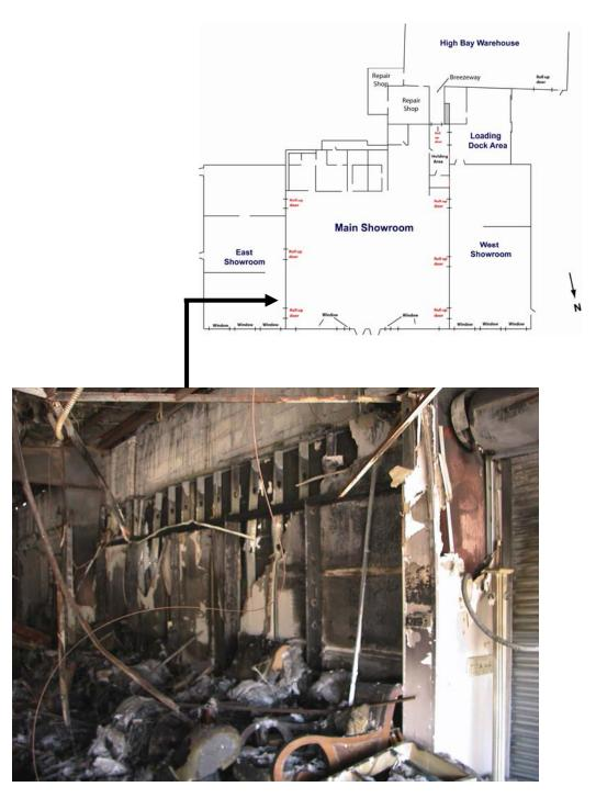
Figure F-19. Interior of east showroom. Closed roll-up fire door visible on right of image.
