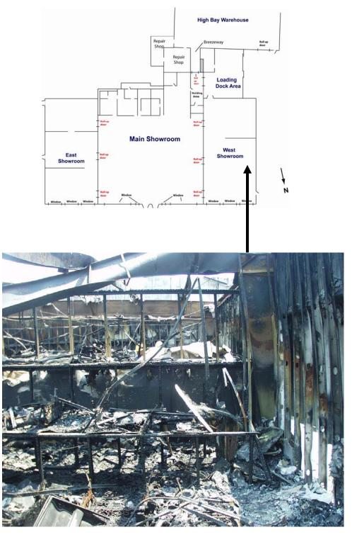
Figure E-18. Interior view along west wall of west showroom. Wood supports for two level display platforms visible in center of photo. Vertical wood studs of partition wall visible behind display platform remnants. Steel I-beam column and roof support also visible on right and top of photo.
