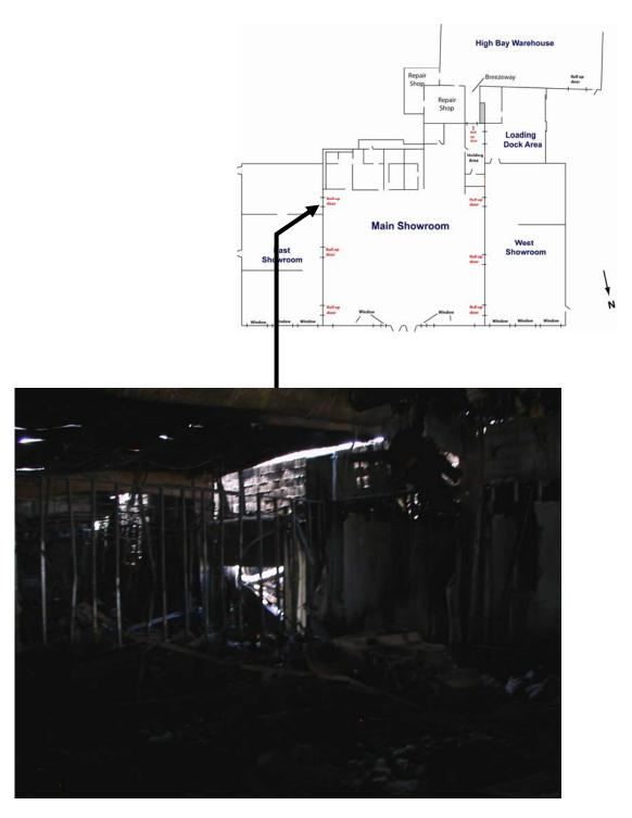
Figure F-16. Interior view of east showroom looking toward partially closed roll-up fire door. Metal studs of rear partition wall visible in left-center background of photo.
