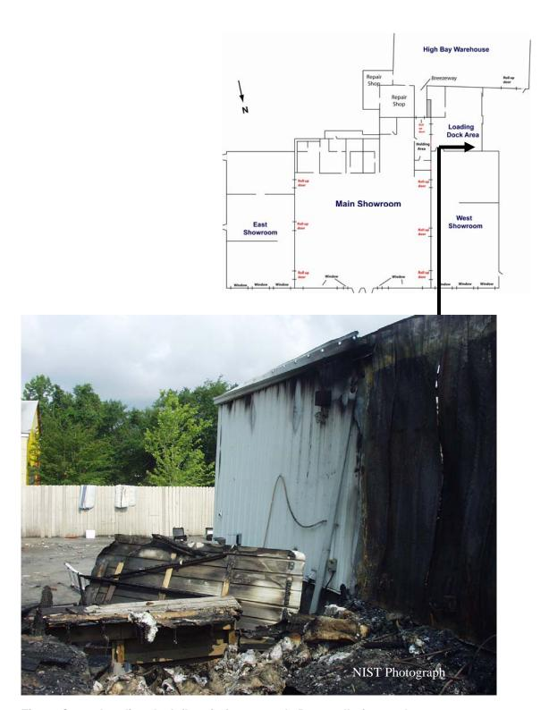
Figure C-16. Loading dock floor in foreground. Rear wall of west showroom on right of photograph. Darker section of rear wall was inside the enclosed loading dock area. Lighter portion of wall was outside enclosed loading dock.
