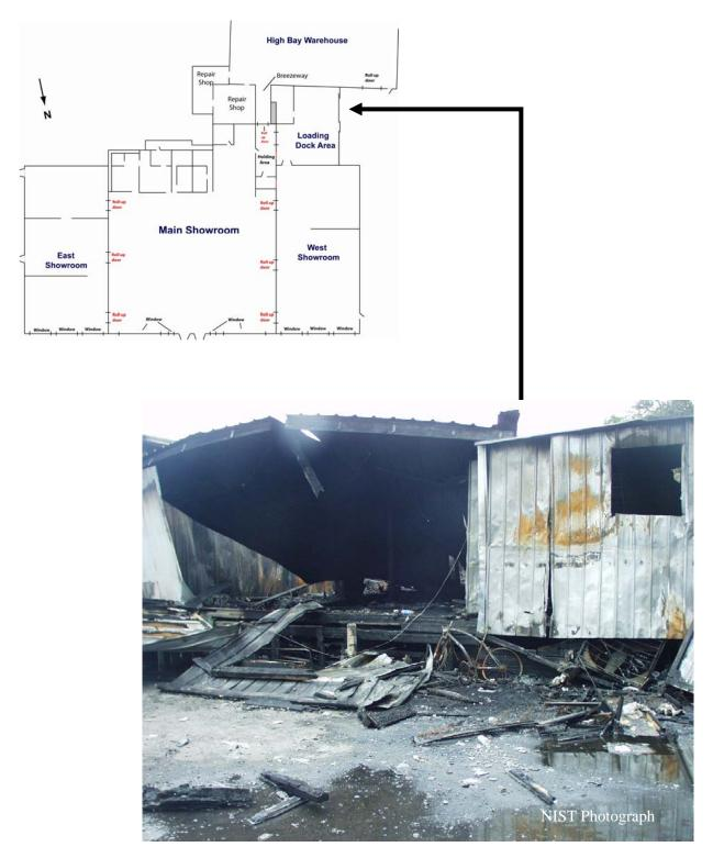
Figure C-5. Left center portion of west wall of loading dock.
