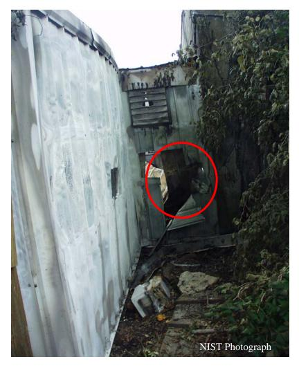
Figure H-3. Intersection of walls of two repair shops with rear wall of main showroom. Trapped employee was extracted from opening in metal siding visible in center of photo (circled area). Air conditioner which had been mounted in rectangular opening in wall fell out and was on ground below opening.
