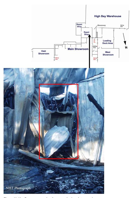
Figure H-13. Doorway opening from repair shop into warehouse.
