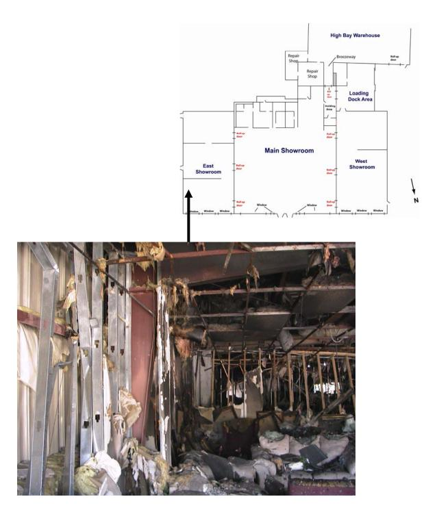
Figure F-21. Interior of east showroom looking along east wall toward rear of showroom. Exterior metal wall attached to exterior side of horizontal channel. Metal studs attached to inside face of horizontal channel. Gypsum wall board was installed over metal studes to form interior wall of showroom. Metal stud/gypsum wall appeared to extend approximately 0.3 m (1 ft) above drop ceiling along east wall. Reddish-brown steel I-beam column and roof joist also visible in photo.
