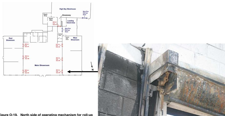
Figure O-19. North side of operating mechanism for roll-up fire door #4. Portion of fusible link visible in center-bottom of photo.
