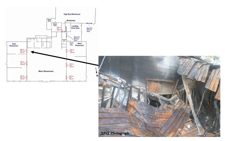
Figure O-55. Main showroom roll-up fire door looking toward rear of east showroom. Door identified as roll-up fire door #7 in Figure O-1. Door only closed about one-third of the way down during the fire.
