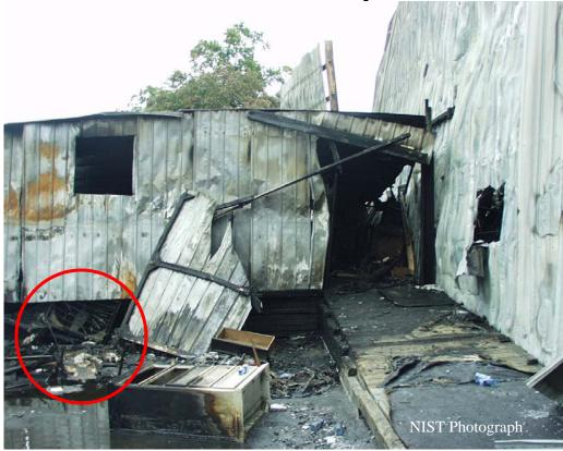
Figure C-4. Right side of west wall of loading dock. Inclined ramp led from warehouse loading dock. Fire ignited in pile of trash outside loading dock (within red circle).
