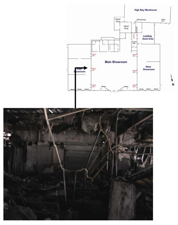
Figure F-15. Interior of east showroom looking toward main showroom. Closed roll-up fire door visible in center of photo. Photo displays more damage from fire in this center section of east showroom.
