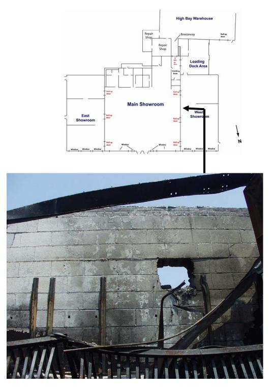
Figure E-26. Interior of west showroom above drop ceiling looking toward main showroom. Open hole, approximately  $0.5 \, \text{m}$  (  $1.5 \, \text{ft}$ ) x  $0.5 \, \text{m}$  ( $1.5 \, \text{ft}$ ) opening through concrete block wall. This hole may have allowed smoke to move from interstitial space above drop ceiling in main showroom to the interstitial space above the drop ceiling in the west showroom.
