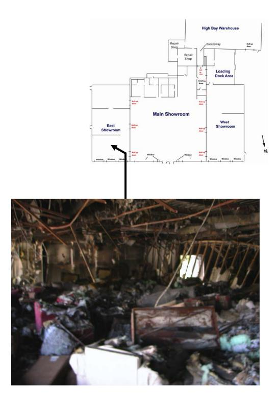
Figure F-12. Interior of east showroom. Wood stud partition wall visible in right background of photo.
