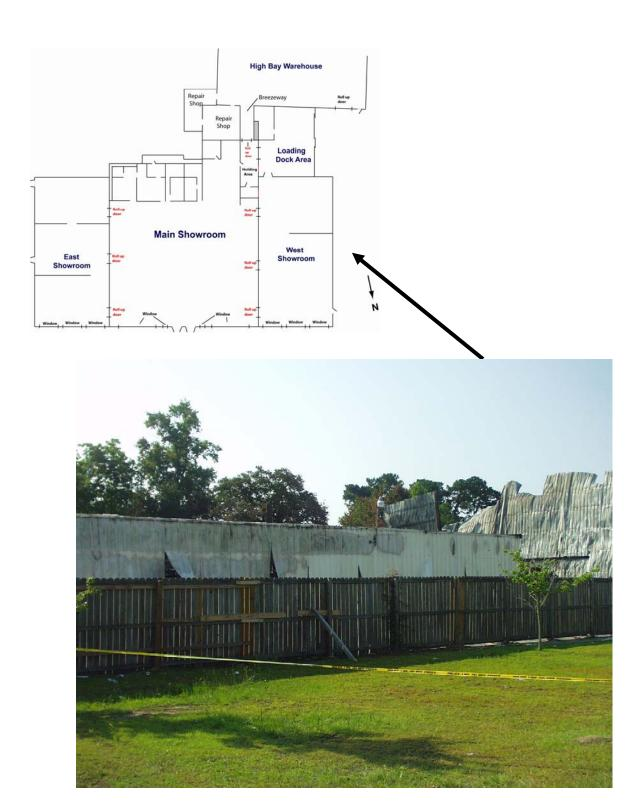
Figure E-6. West wall of west showroom. Discoloration patterns due to exposure to high temperatures visible on metal siding. Front section of west showroom displayed more discoloration than rear section of west showroom. Wooden fence separates furniture store from adjacent property.
