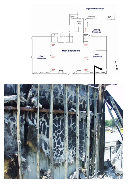
Figure E-31. Interior of west showroom looking at west wall near front of store. Exterior metal wall attached to exterior side of horizontal channel. Metal studs attached to inside face of horizontal channel. Gypsum wall board was installed over metal studs to form interior wall. Metal stud/gypsum wall appeared to extend approximately 0.3 m (1 ft) above drop ceiling along west wall. Fiberglass insulation is visible between metal studs and exterior metal siding.
