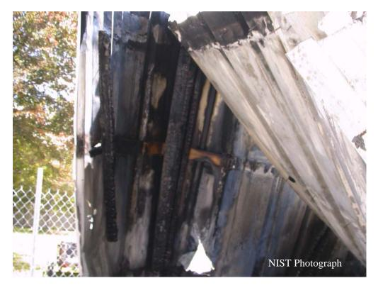
Figure H-6. Wood frame of repair shop.
