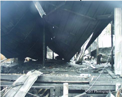
Figure C-3. Remains of center portion of west wall of loading dock. Line of studs on right supported 2.7 m (9 ft) high section while line of studs in left center of image supported 3.7 m(12 ft) high section.
