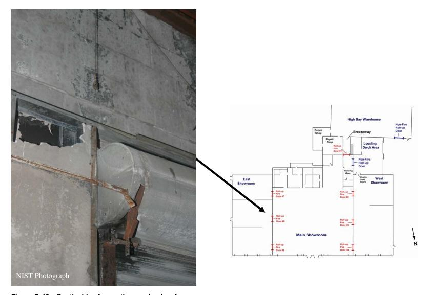
Figure O-46. South side of operating mechanism for roll-up fire door #6. Portion of fusible link visible in center of photo.
