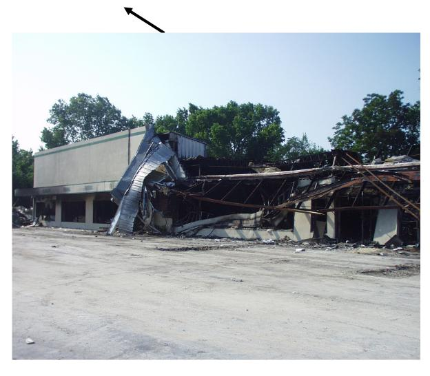
Figure D-13. Front of main showroom after removal of collapsed façade. Façade and parapet wall of east showroom still in place.
