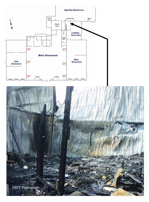
Figure C-11. Rear wall of loading dock area/metal breezeway wall intersect with north wall of warehouse.
