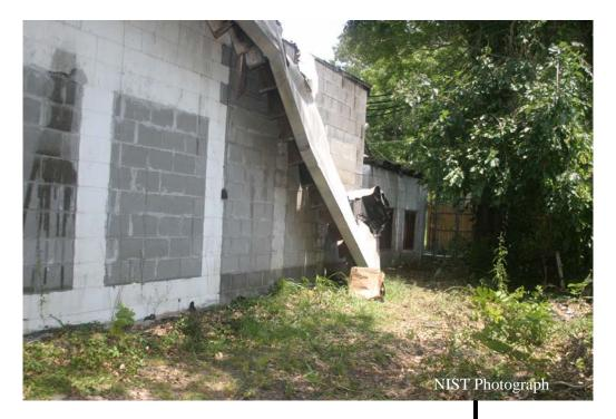
Figure I-7. Rear wall of main showroom. Openings in wall have been filled with concrete block. Wood fence visible in center right of photograph.
