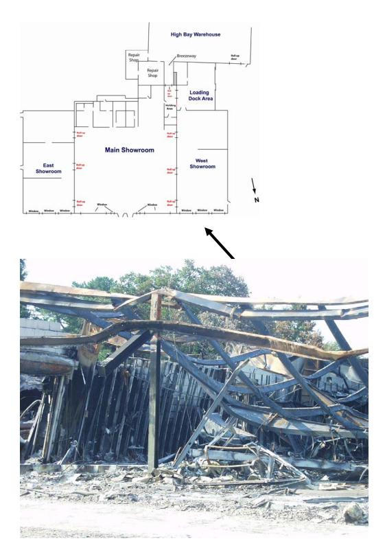
Figure E-13. Exterior view of west showroom looking into east-front portion of showroom. Metal stud wall attached to west wall of main showroom visible in center of photo. Open roll-up fire door partially visible at left center of photo.
