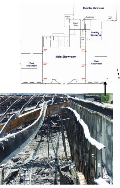
Figure E-16. Interior view of west showroom at top of exterior wall. View looking into showroom toward rear of showroom.
