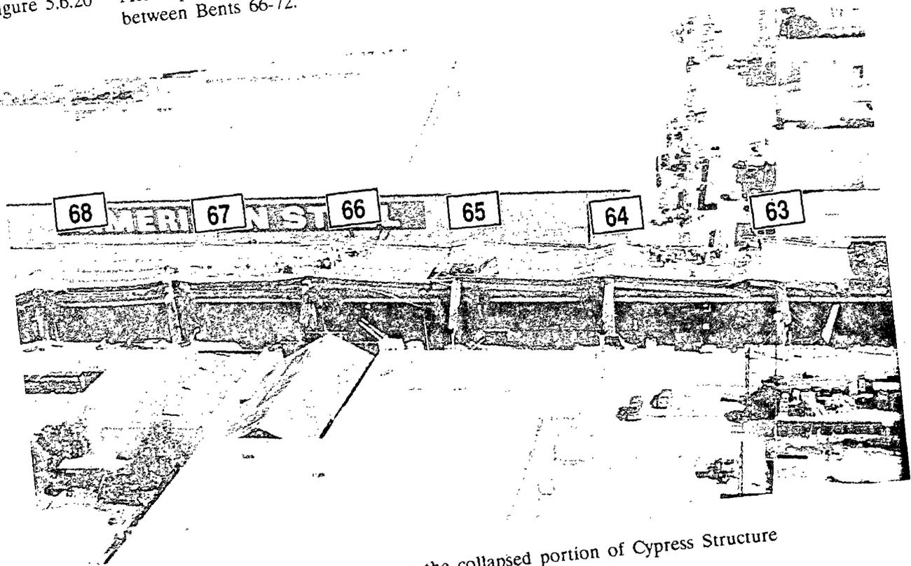
Figure 5.6.21 Aerial photo looking east to the collapsed portion of Cypress Structure between Bents 62-68.
