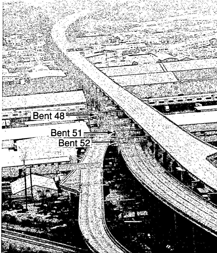
Figure 5.9.2 Aerial view of I-280 south of Army St., note the transition from a two-level elevated structure to a single-level, divided structure (view is looking south).
