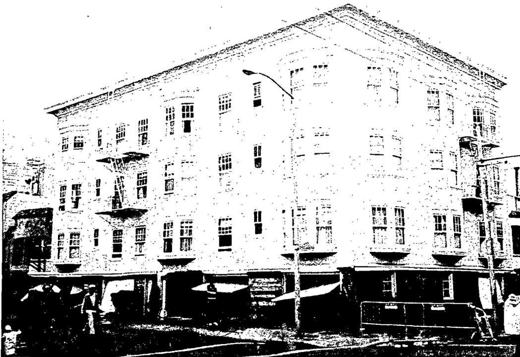
Figure 4.2.13 Example of four-story building with multiple garages in the first story (location #9).
