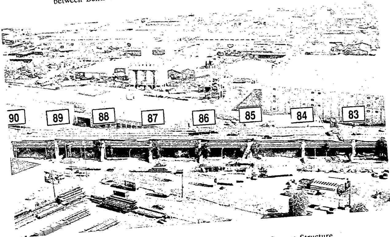
Figure 5.6.17 Aerial photo looking east to the collapsed portion of Cypress Structure between Bents 83-90.
