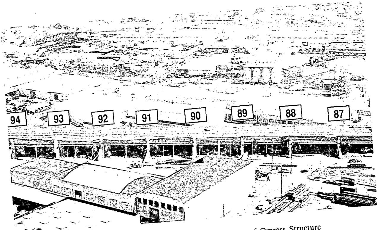
Figure 5.6.16 Aerial photo looking east to the collapsed portion of Cypress Structure between Bents 86-94.
