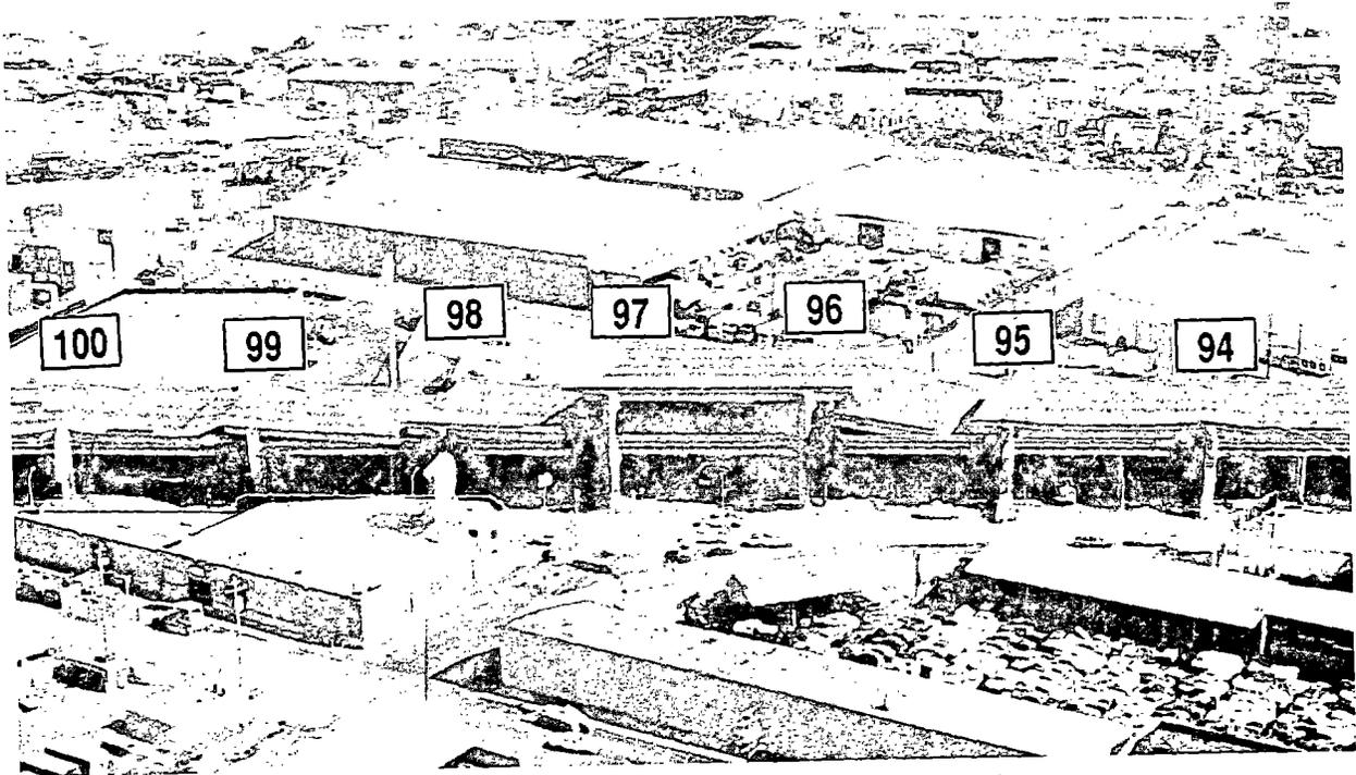
Figure 5.6.14 Aerial photo looking east to the collapsed portion of Cypress Structure between Bents 94-100.
