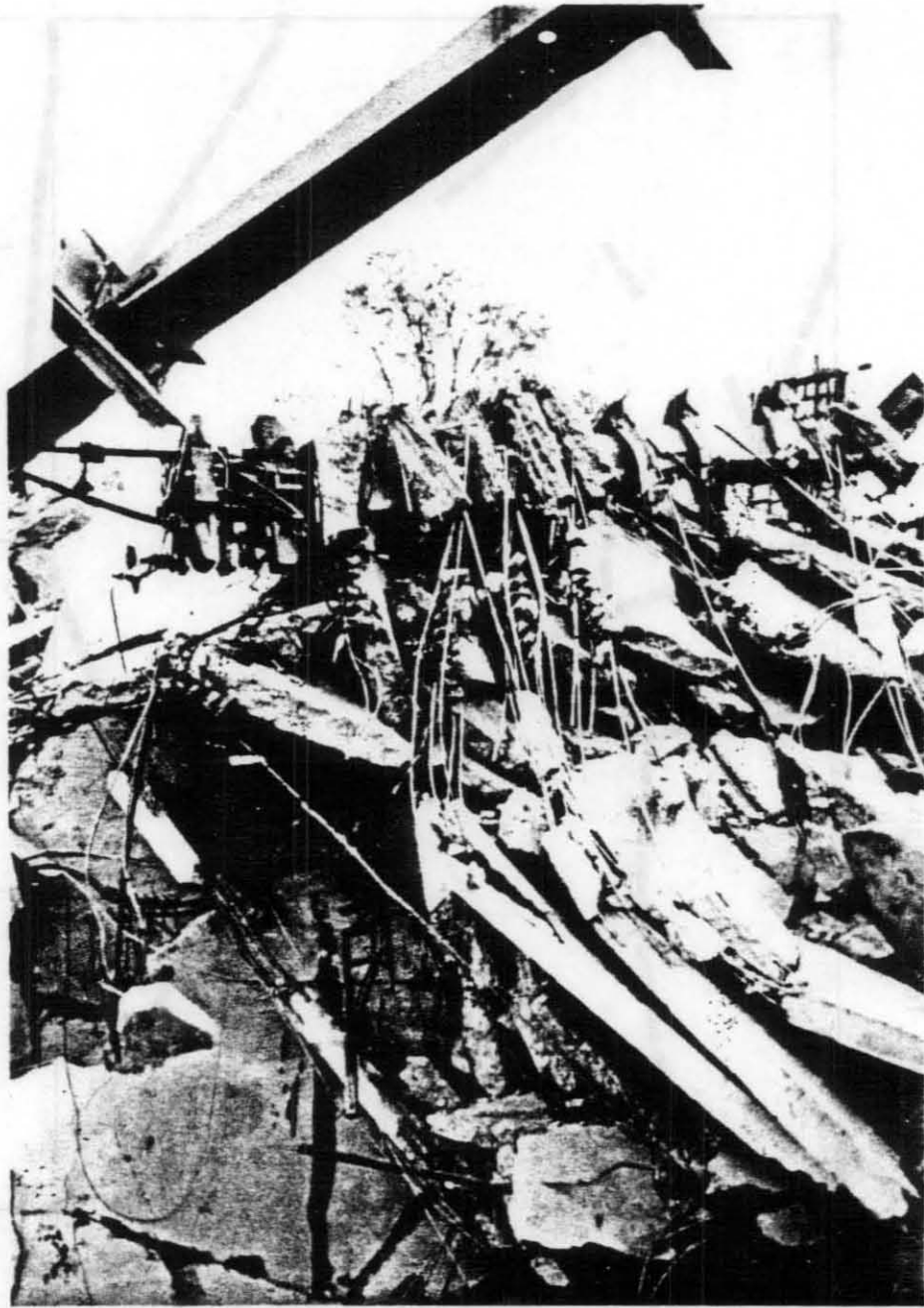
Figure 4.4.15 Separation of floor slabs from shearheads
