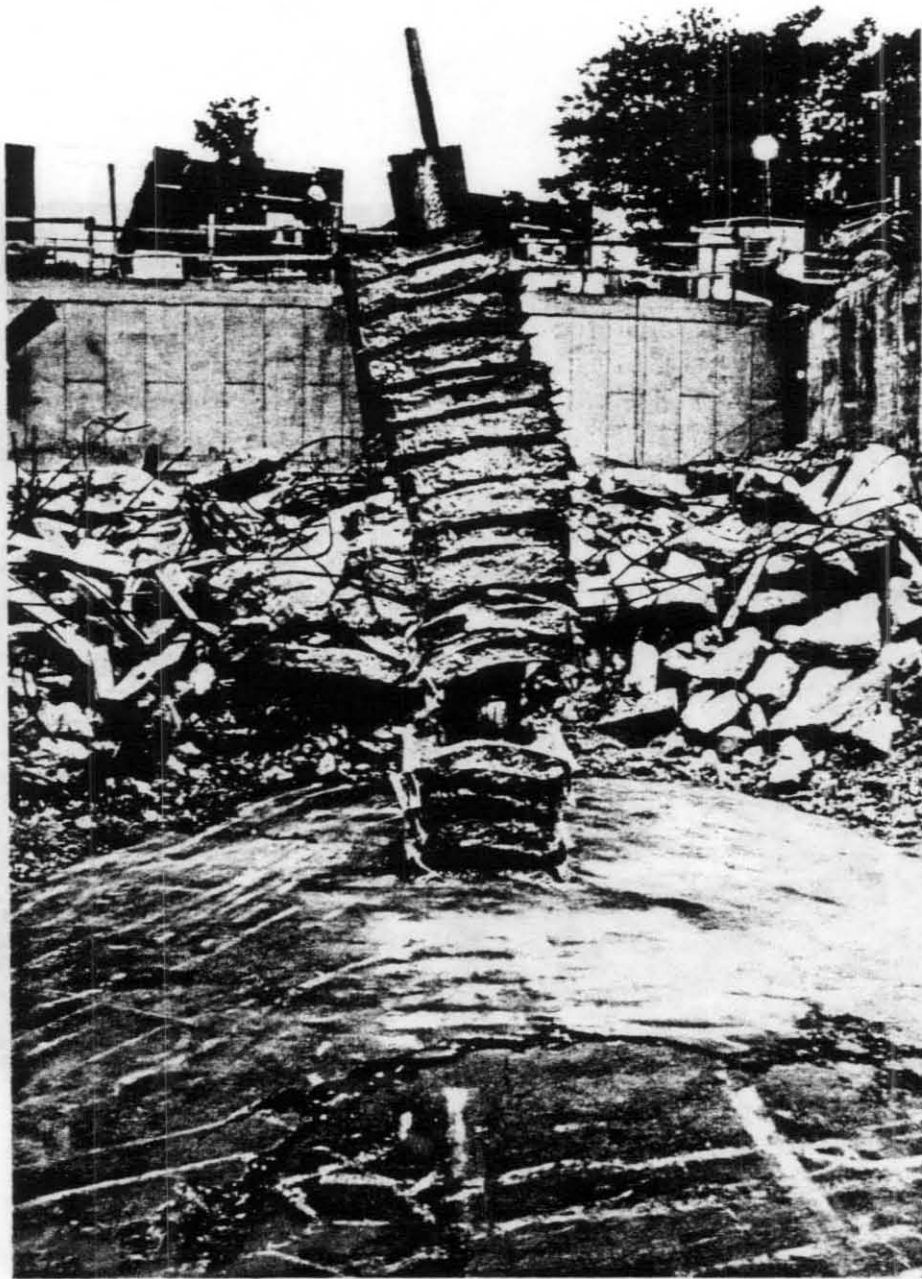
Figure 4.4.18 Deformation pattern of shearheads – column D10
