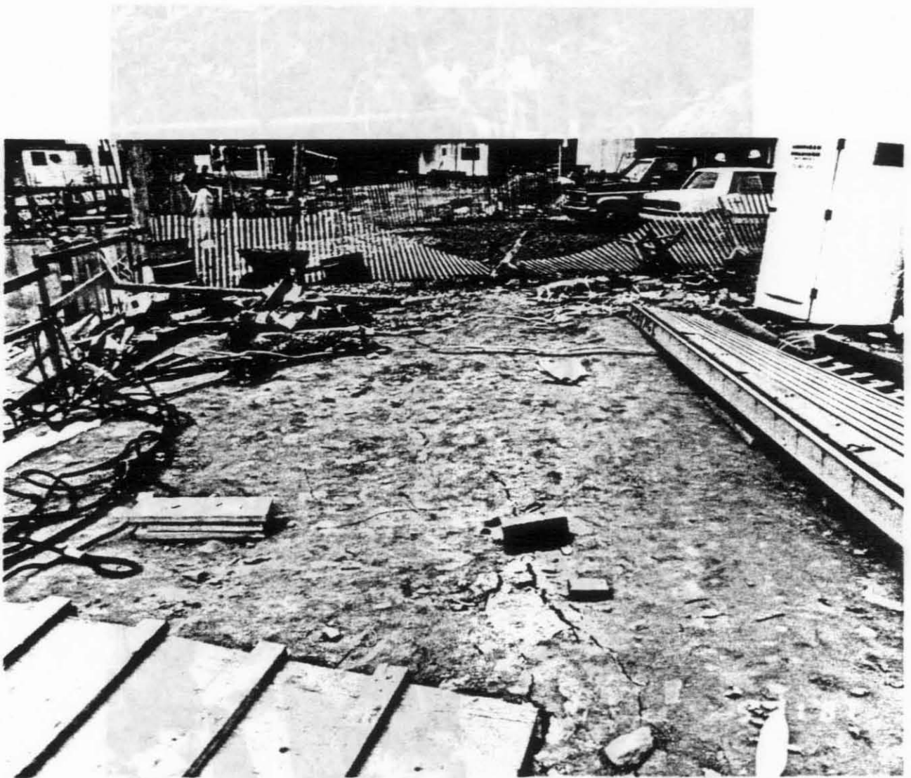
Figure 4.4.31 Tension cracks in backfill behind basement wall – North side of building
