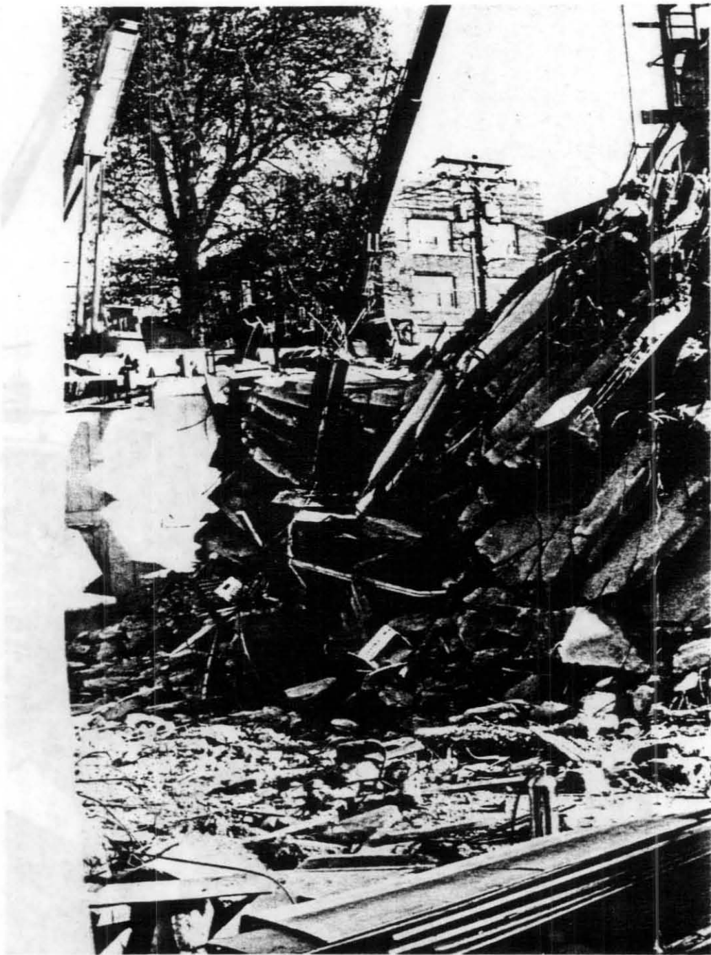
Figure 4.4.8 Lower level floor slabs at Northwest corner of West tower – View to the North; column E1
