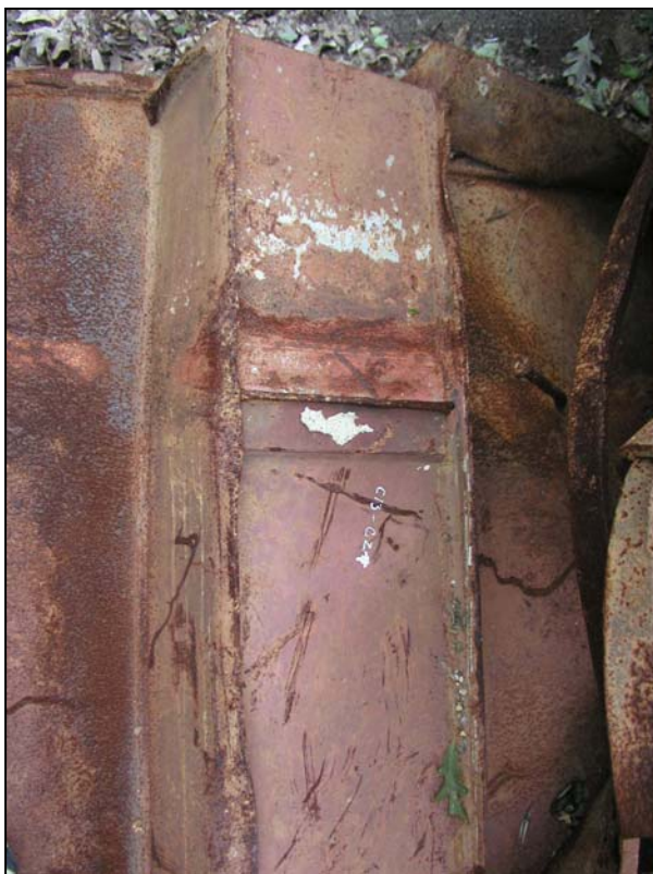
Figure A3c: Type C floor truss connector
