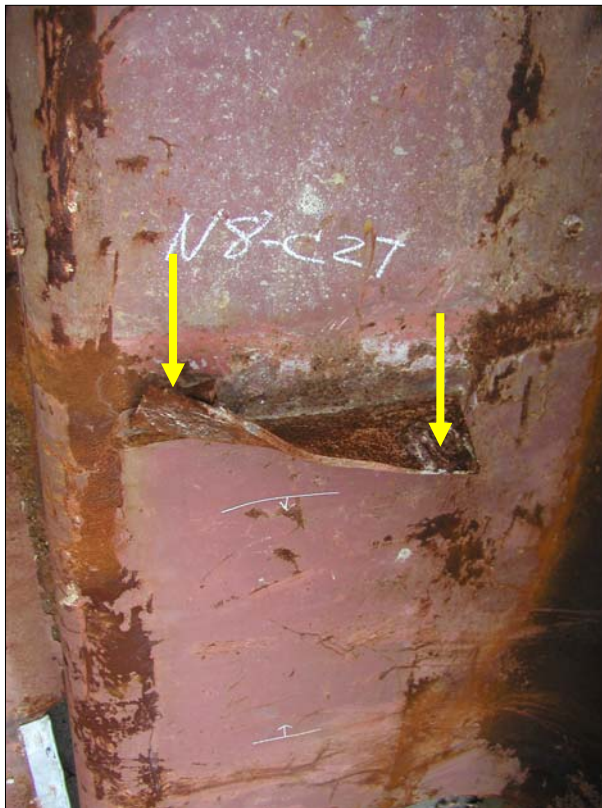
Figure A3a: Type C floor truss connector
