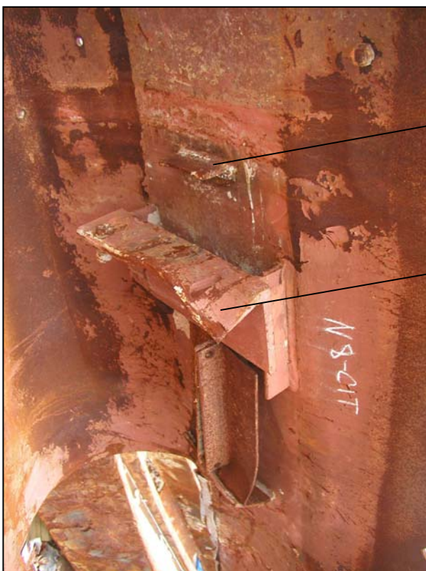
Figure A1a: Type A floor truss connector
