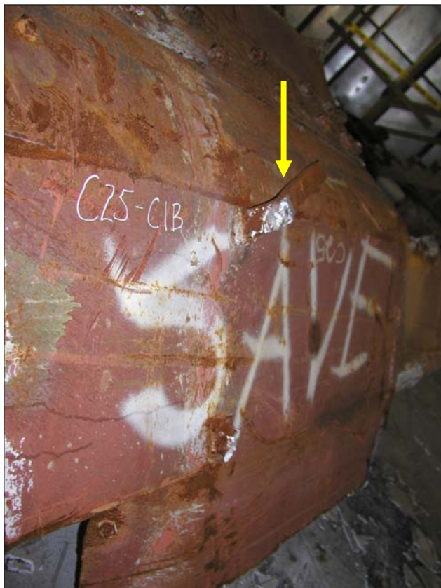
Figure A4a: Type D floor truss connector
