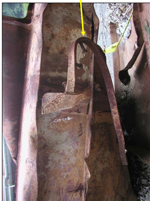
Figure A3d: Type C floor truss connector
