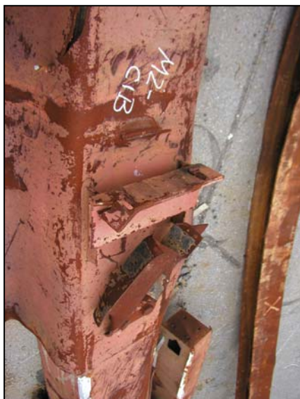
Figure 6–27. Floor truss connectors for panel M-2 (A130: 96-99).
