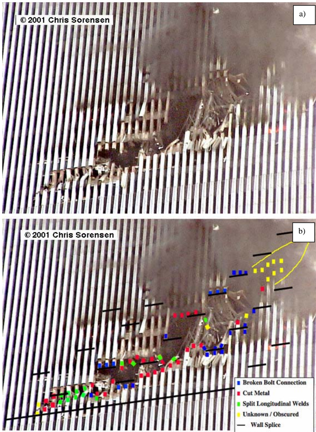
Figure 6-2. (top) Enhanced image showing the impact hole in the south face of WTC 2 and (bottom) overlay of the location and type of localized damage.
