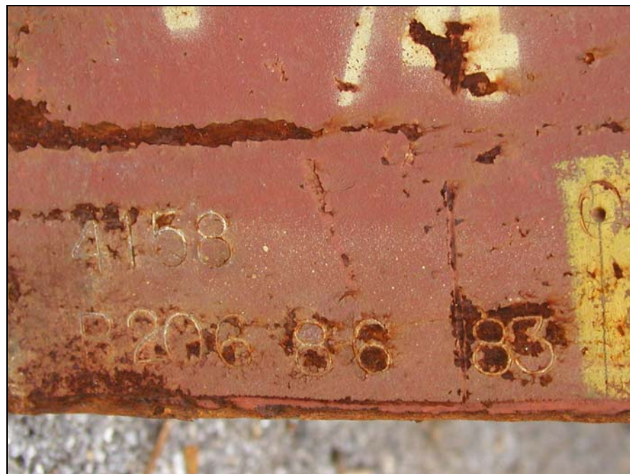
Figure 5–1. Example of stampings on the interior base of the middle column for each panel. Shown here on panel M-10b are the stampings “B206 86 83,” indicating that it is from WTC 2, column number 206, spanning floors 83 to 86.
