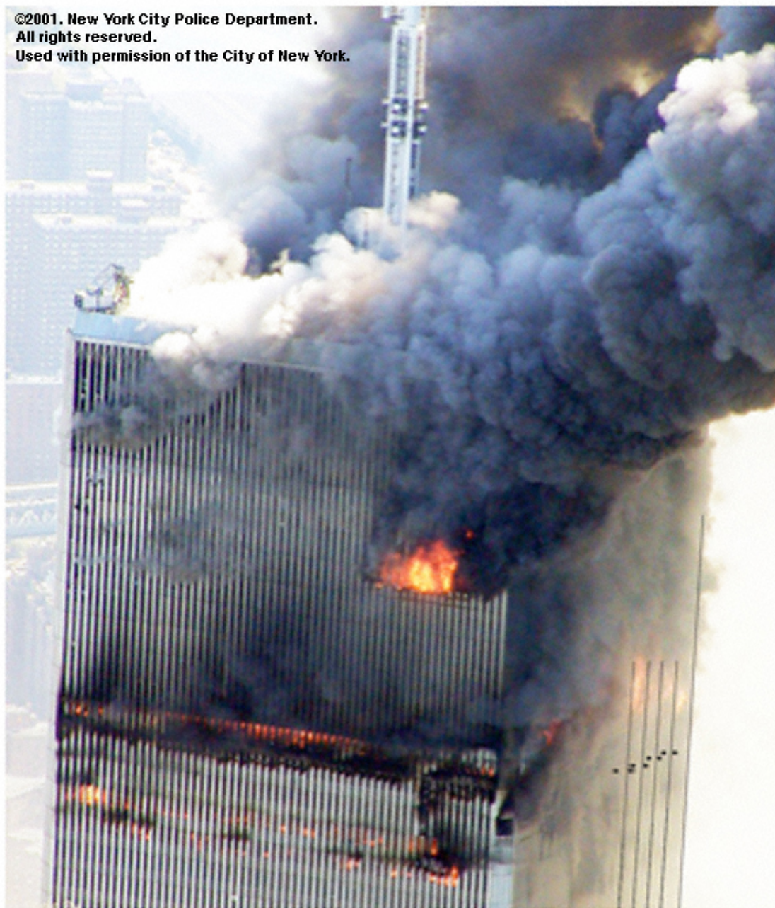
Figure 6–14. Inward bowing of south face (at right, with dark lines overdrawn) of WTC 1. Taken at 10:23 a.m. from an NYPD helicopter.
