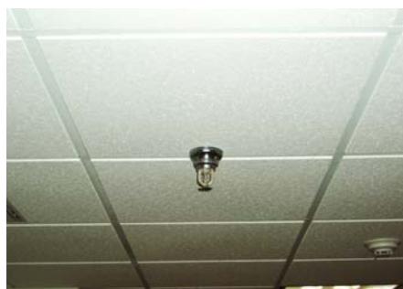
Figure 3–1. Typical sprinkler installed in ceiling.
