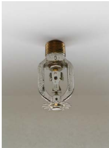
Figure 5–11. Typical standard spray pendent sprinkler.
