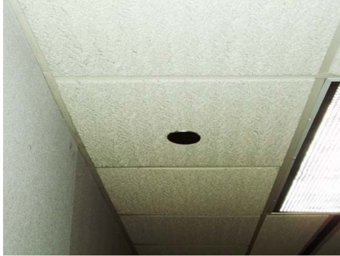
Figure 5–10. Typical concealed pendent sprinkler.
