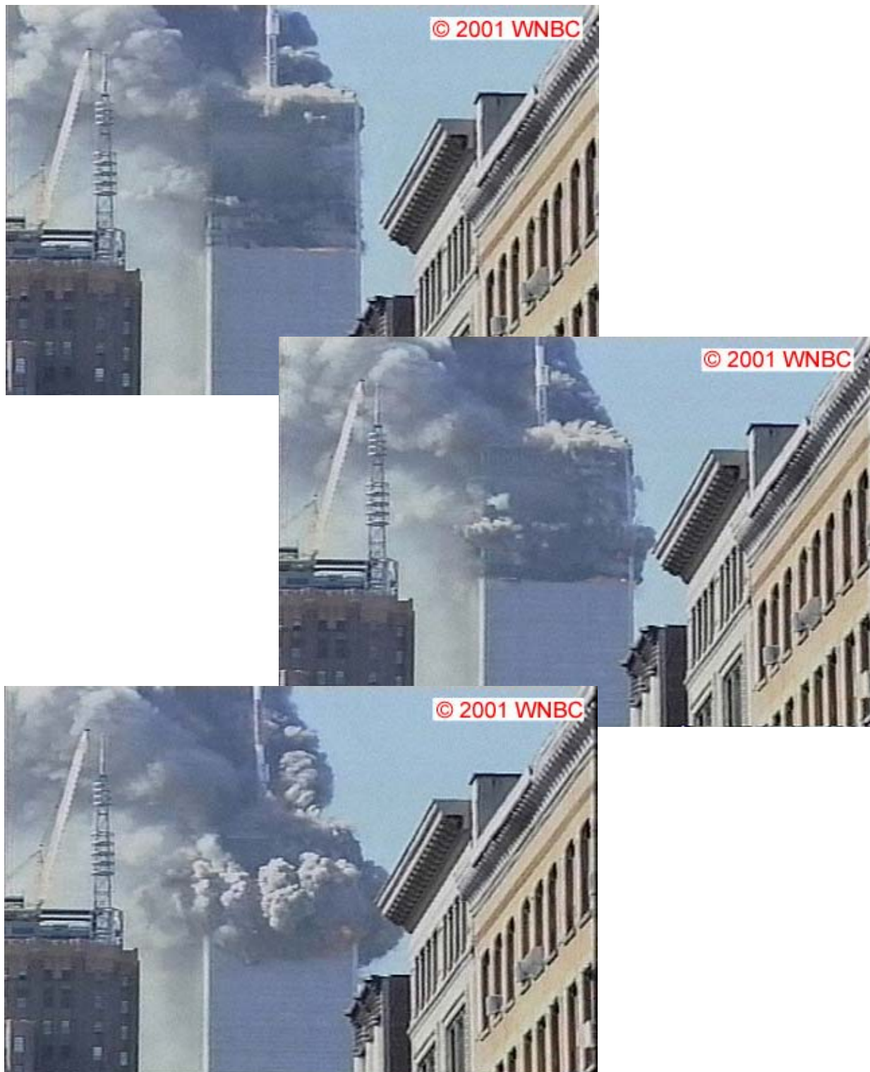
Figure 6–10. Rotation of WTC 1 building section above the aircraft impact zone toward the south as viewed from due north. Note that there is no tilt in the east or west directions.
