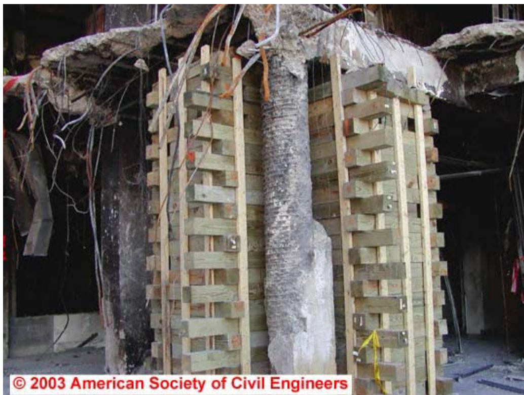
Figure 5–27. Typical damage to spirally reinforced columns in the Pentagon not impacted or bent by large debris (ASCE, 2003).
