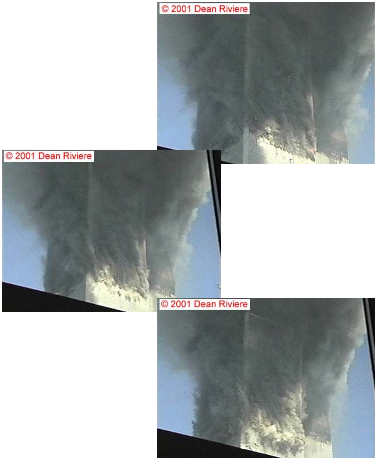
Figure 6–23. View of east wall buckling and WTC 2 collapse from southeast.
