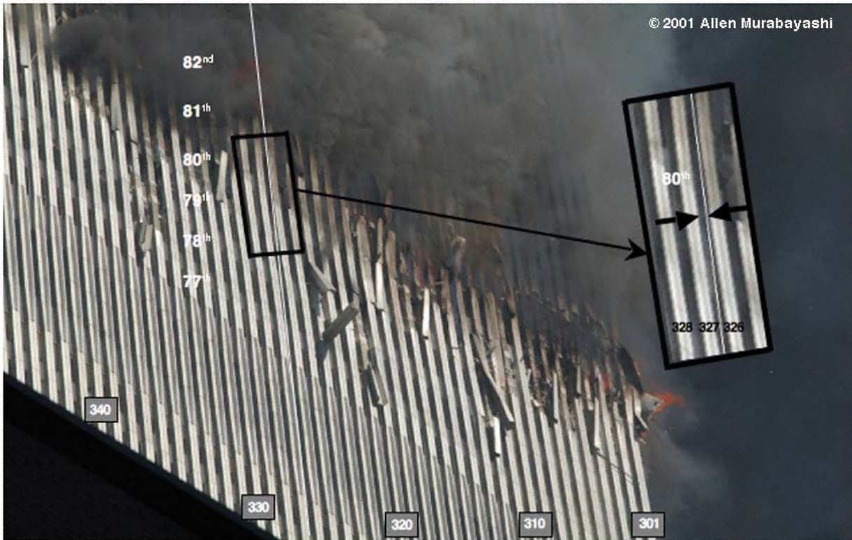
Figure 6-17. WTC 2 exterior columns bowing inward across north side of the east face between Floors 77 to 83 at 9:21 a.m.
