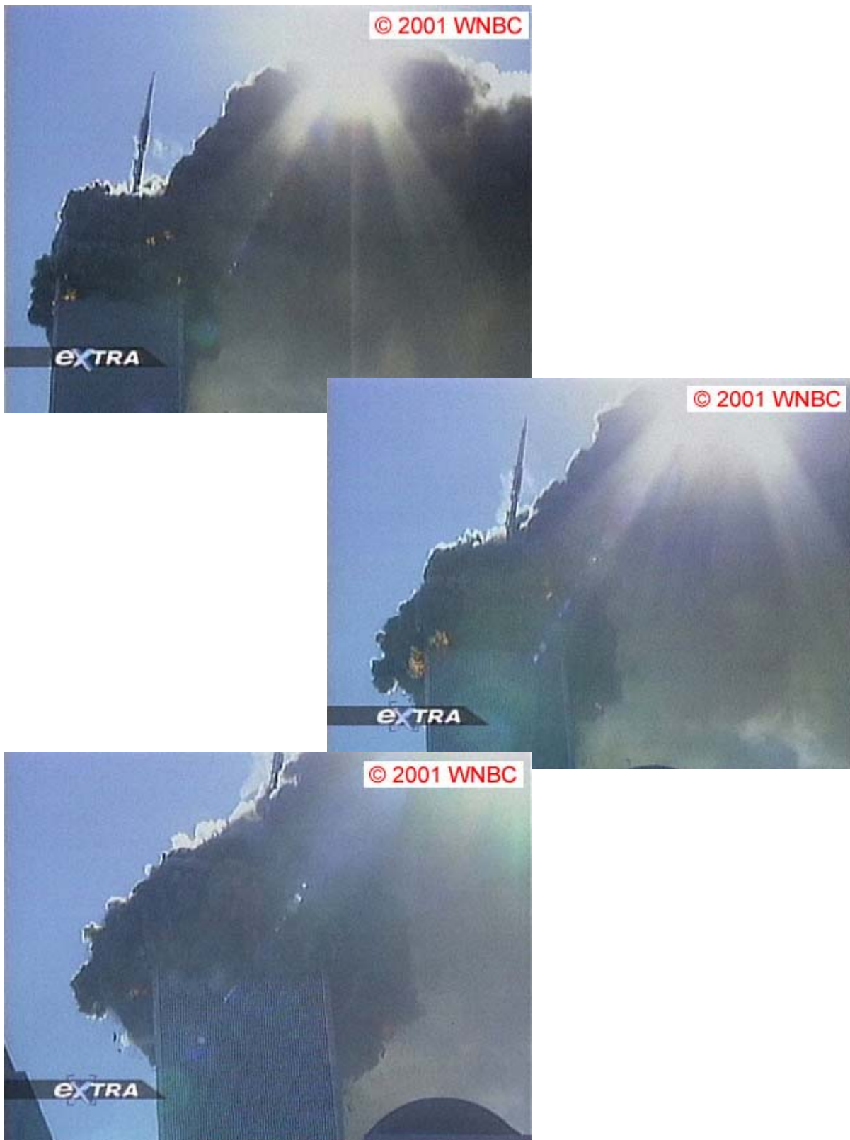
Figure 6–11. WTC 1 tilt to the south of approximately 8 degrees was measured before smoke and debris obscured view. Note view is from west and tilt is directly south.
