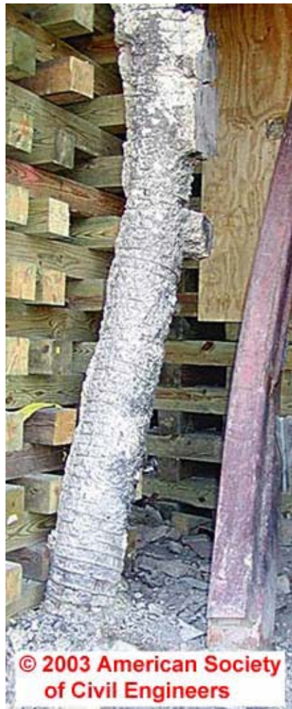
Figure 5–26. Typical damage to spirally reinforced columns in the Pentagon impacted and bent by large debris (ASCE, 2003).
