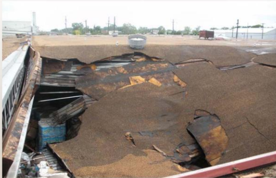
Rain/drainage: soaked cover boards and ponding
