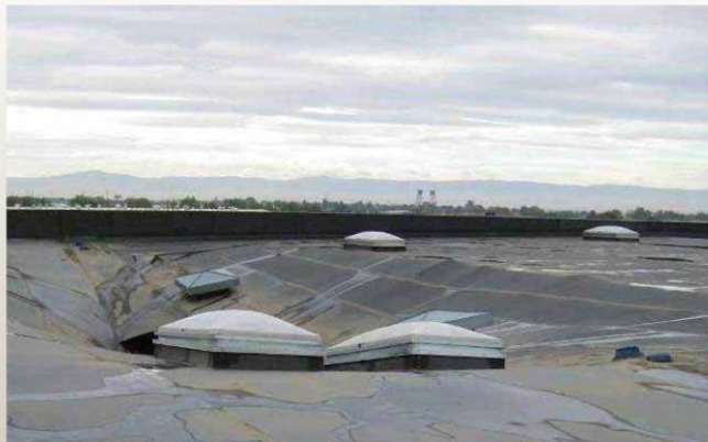
Partially blocked drains, slope
