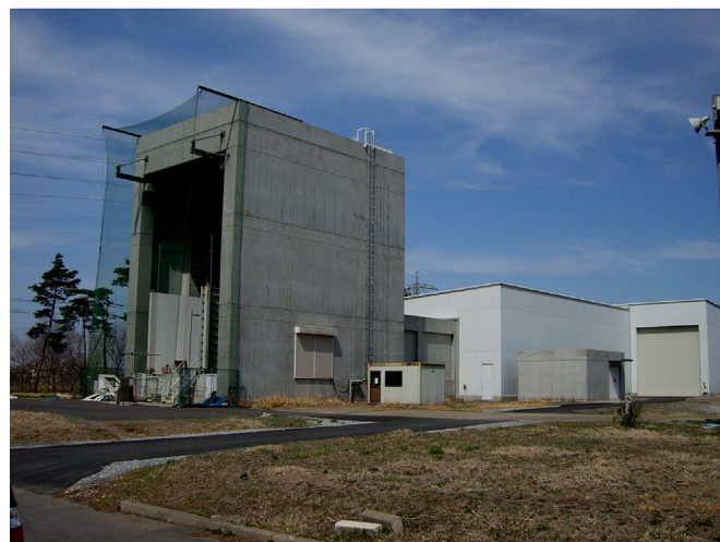
Fig. 3. Overview of Experimental Facilities at the Building Research Institute (BRI). (Fire Research Wind Tunnel Facility (FRWTF), Wind Speeds Up to 10 m/s, Wind Cross-Section: 4.0 m (High) by 5.0 m (Wide), Test Section Length: 15.0 m).
