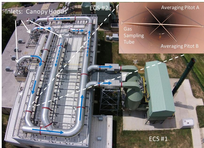
**Fig. 1.** Overhead view of the National Fire Research Laboratory, its rooftop exhaust ducts, flow measurement location, and emissions control systems (ECSs). Blue arrows mark flow paths from the canopy hoods to the two ECSs. Solid arrows mark the flow path of the present study. Dotted arrows mark flow paths for the other canopy hoods and/or the second ECS. The averaging pitot tubes and the gas sampling tube are shown in the insert.
