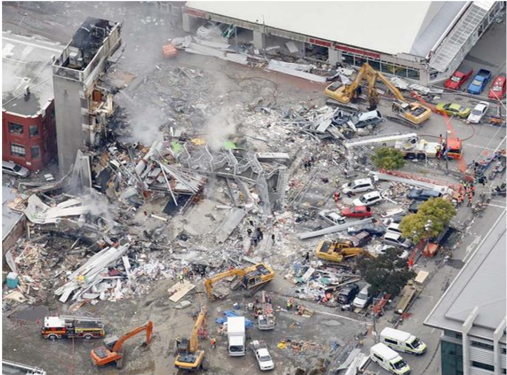
Figure 2-2 CTV Building earthquake damage (New Zealand Herald, 2011).
