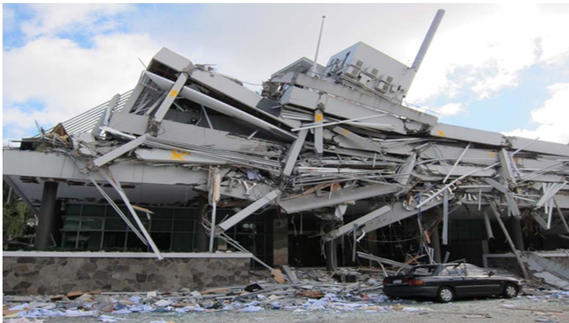
Figure 2-8 Pyne Gould Building earthquake damage (Elwood, 2011).
